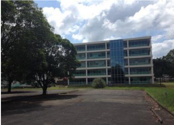
Figure 3. Existing industrial building
